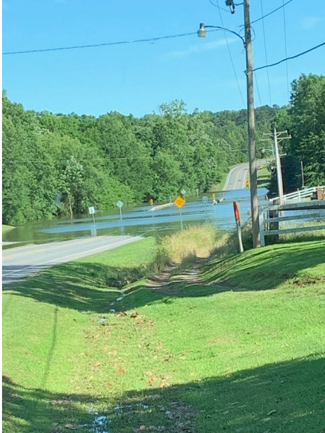
Flooding on Hwy 25 South at Wooster looking south, Greenbrier Creek
